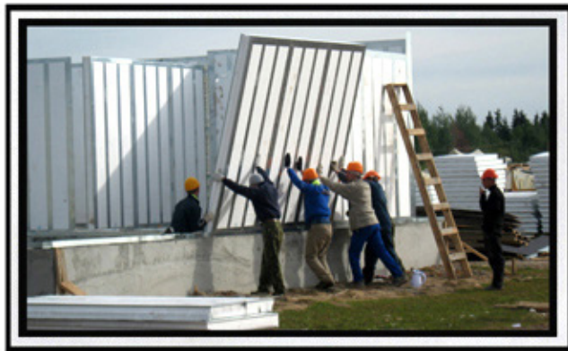
No heavy equipment needed to place panels
